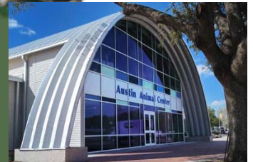
Animal Services Center Status: Post-Construction, p.8
