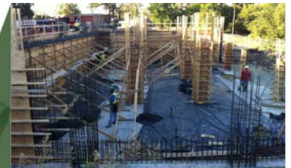
EMS Mueller Station #33 Status: Construction, p.7
