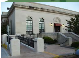
Exterior Renovations Status: Post-Construction, p.6
