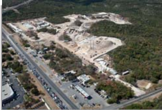
Water Treatment Plant 4 Status: Construction, p.12
