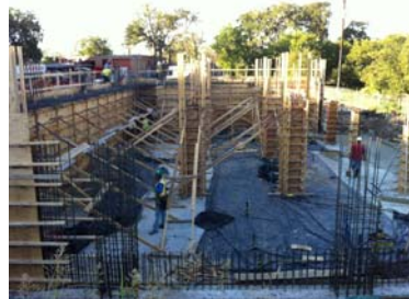
Figure 4. Construction of Station 33
