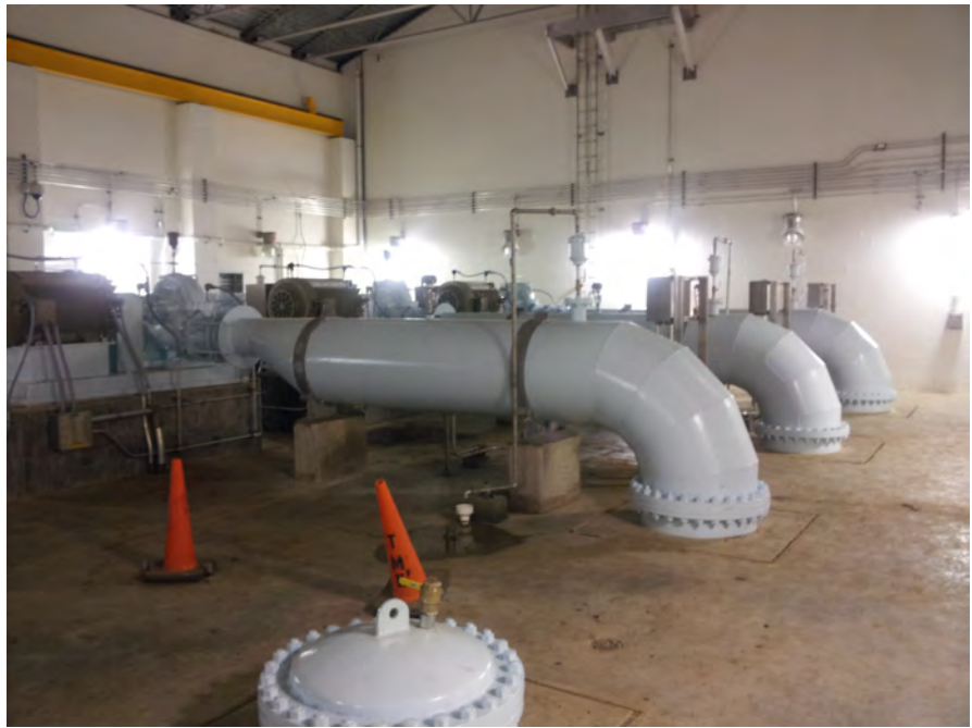
(Above) Motors and pumps in the Pilot Knob Pump Station used to deliver potable water. (Below) The Raw Water pump station at Water Treatment Plant 4.
