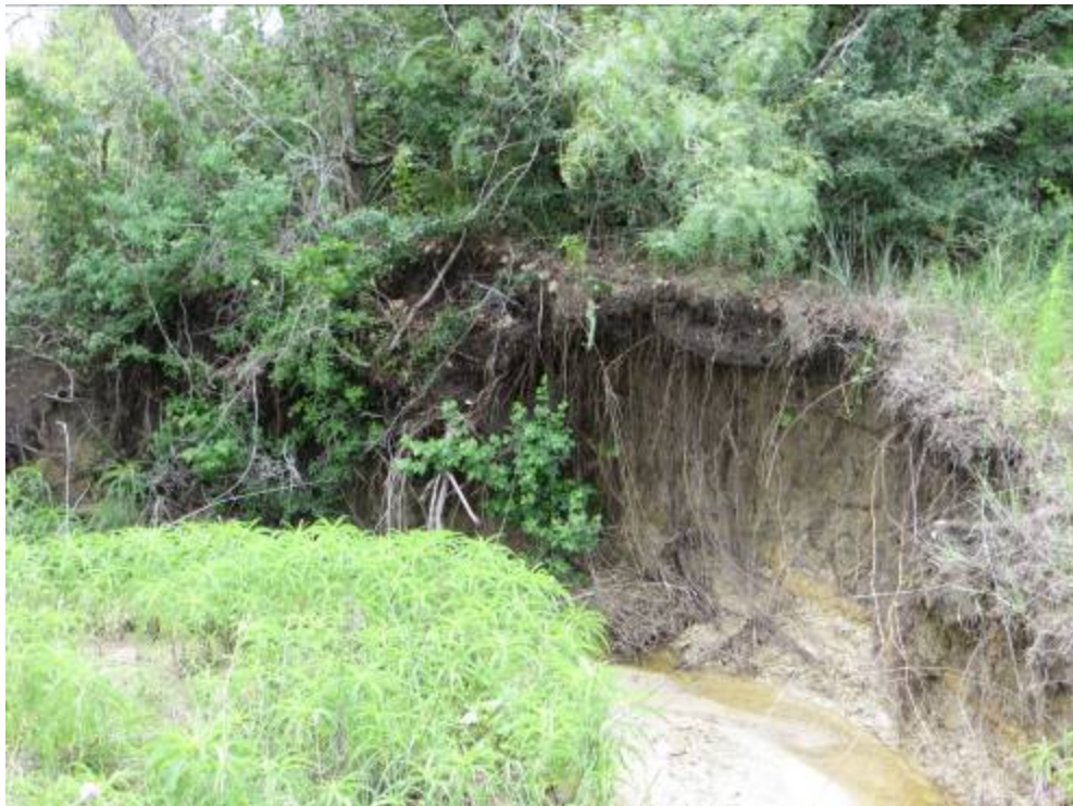
Reach 5.2 Bank Erosion
