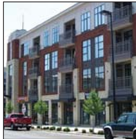
Figure 5-4: Image showing example of building articulation.
