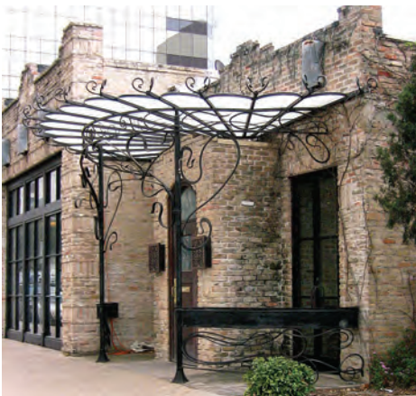
Metal awning and facade created by Mind Over Metal at 311 W. 6th Street
