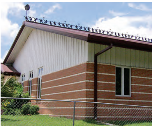
Metal art on roof ridge at 10th St. & Navasota www.fisterrastudio.com/7th.html
