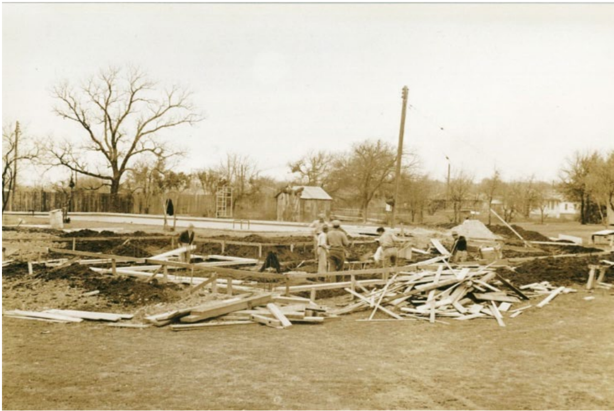
Figure 23. Photo of bathhouse construction dated February 7, 1941. Austin History Center: Austin Files – Parks, P1200(31), Zaragoza.
