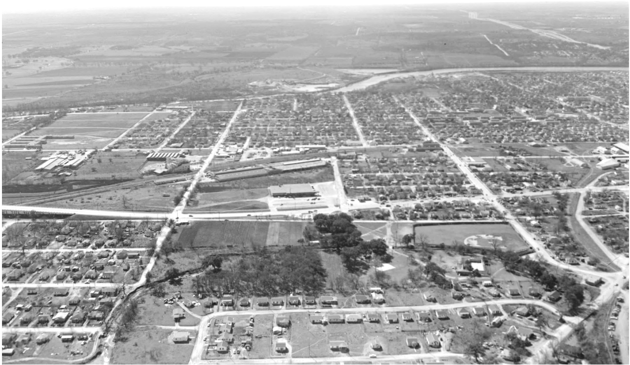
Figure 27. Aerial photo looking south from East Austin, dated January 11, 1958. Parque Zaragoza is in the center-right foreground with baseball diamond and pool/bathhouse. Austin History Center and University of North Texas, Portal to Texas History, https://texashistory.unt.edu/ark:/67531/metaph19192/m1/1/?q=%22zaragoza%20park%22 .
