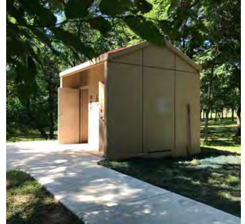
Site Photo: OCOMP
