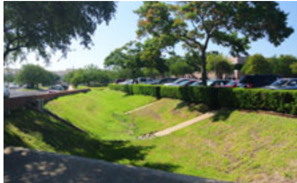
Swales: stormwater management in suburban areas.
