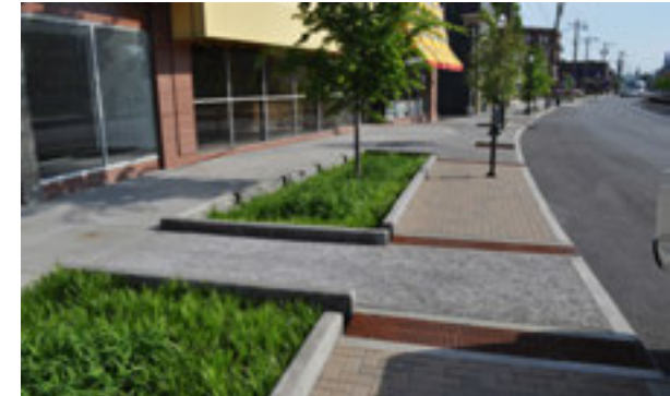
Biofiltration on the sides of streets in an urban area.
