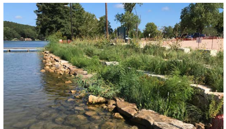
Figure 7. The new shoreline shows that modern methods can provide stability and ecological function in harmony with recreation.
