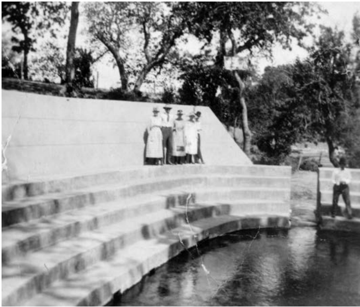
Figure 10. The original configuration of the Eliza amphitheater in 1903. The “keyhole” where water exited between the steps was filled in the late 1920s.
