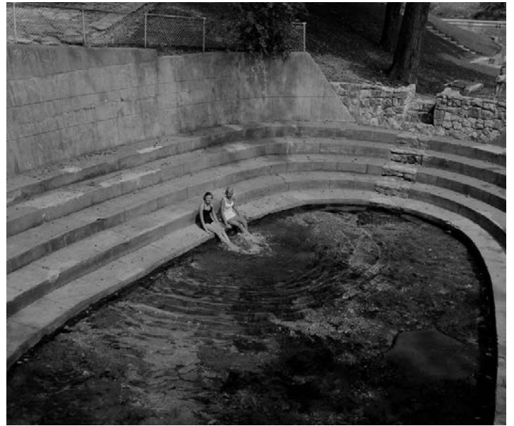
Figure 11. The Eliza Spring amphitheater after the keyhole was filled and stream buried into a pipe
