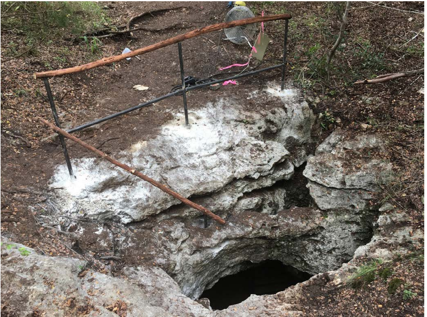
Figure 7. The new handrail and steps make it easier for educational groups to visit Wade Cave's underground habitat.
