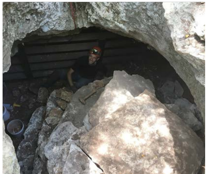
Figure 8. For years before Wade Cave was restored, broken glass and ranch trash filled the entrance. Now the entrance is filled by big limestone steps leading to this underground habitat.
