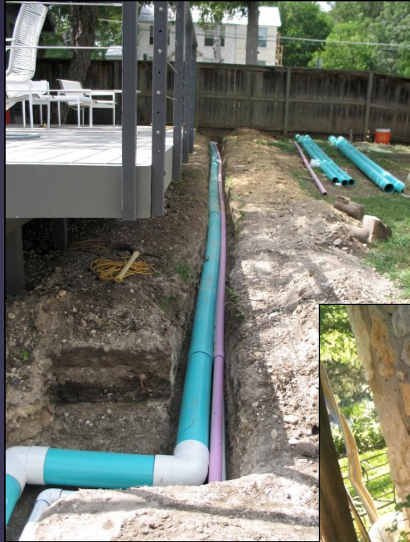
Underground/ downspouts
